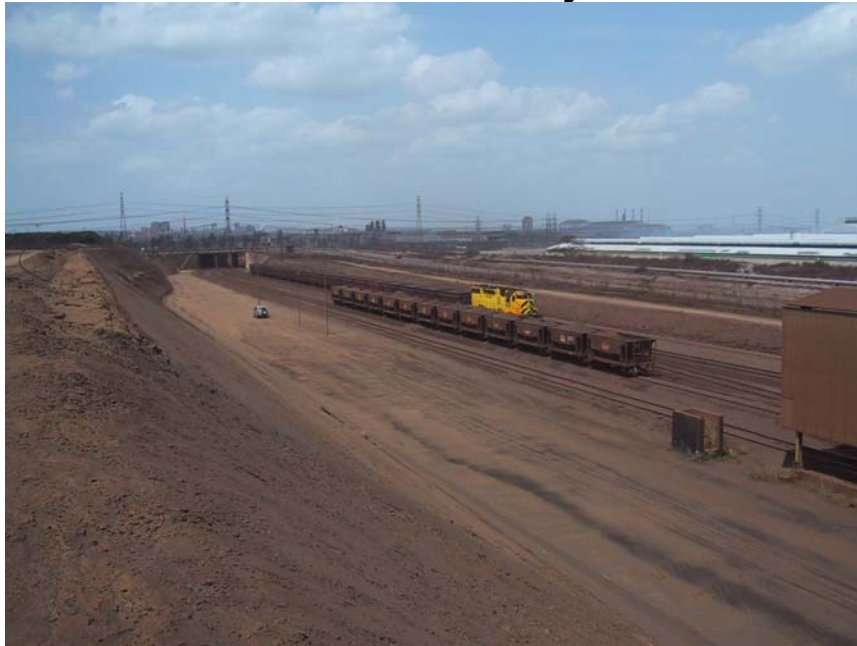
Figure 1 Iron Ore Delivery
