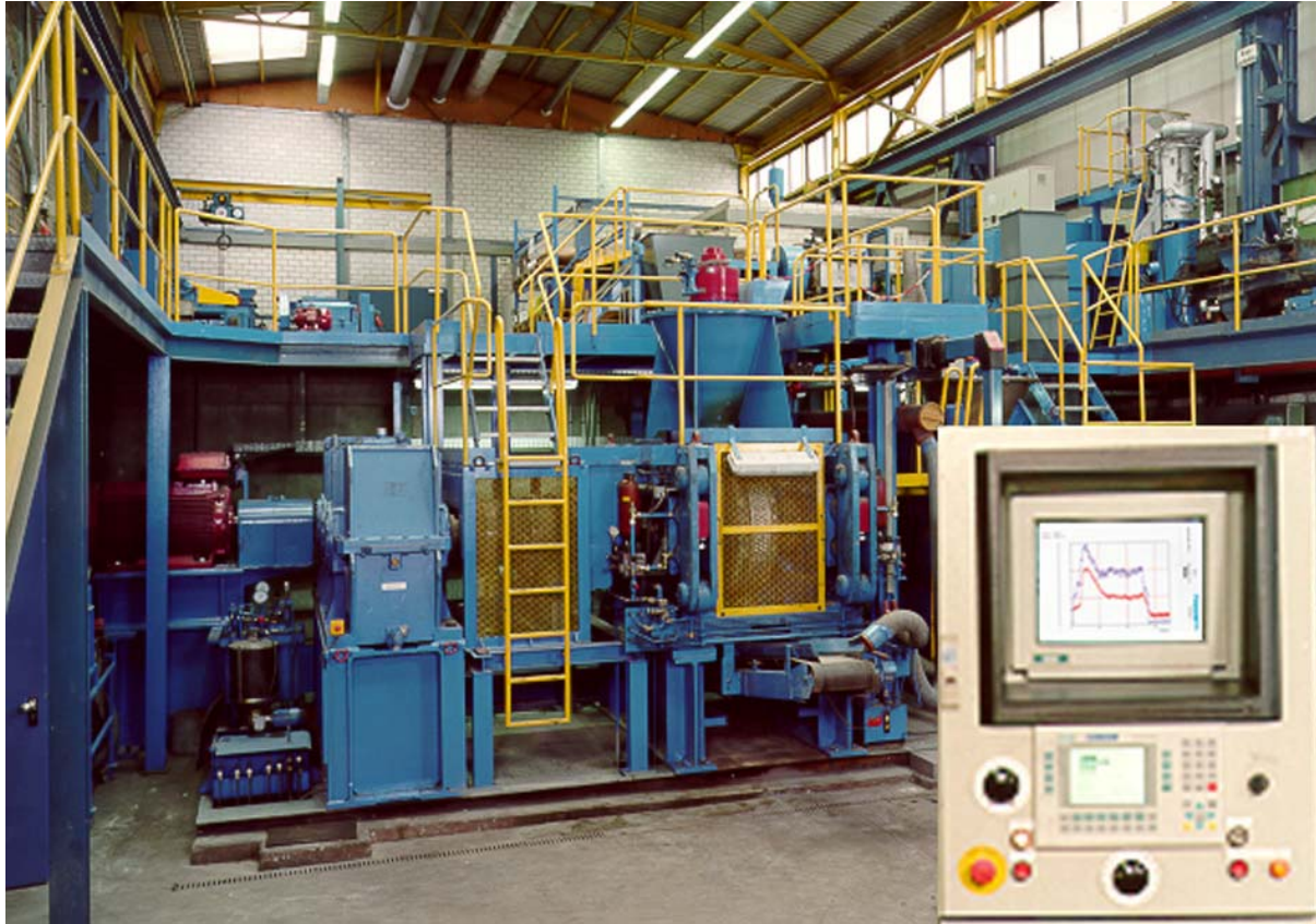
Figure 5: Large scale instrumented roller press at KÖPPER's test facility.
